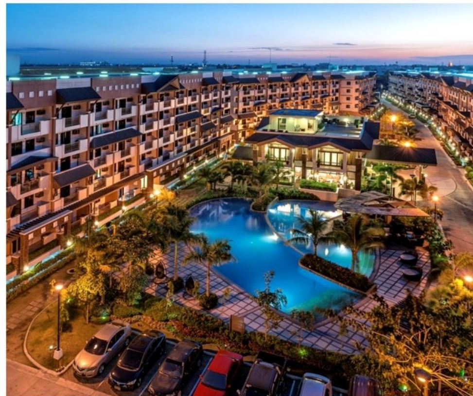
ACTUAL PHOTO OF THE DEVELOPMENT
