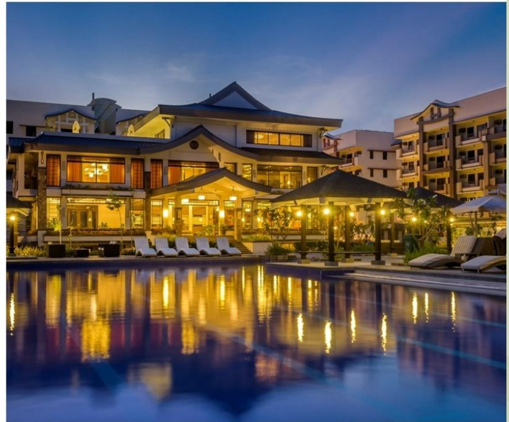
ACTUAL PHOTO OF THE DEVELOPMENT
