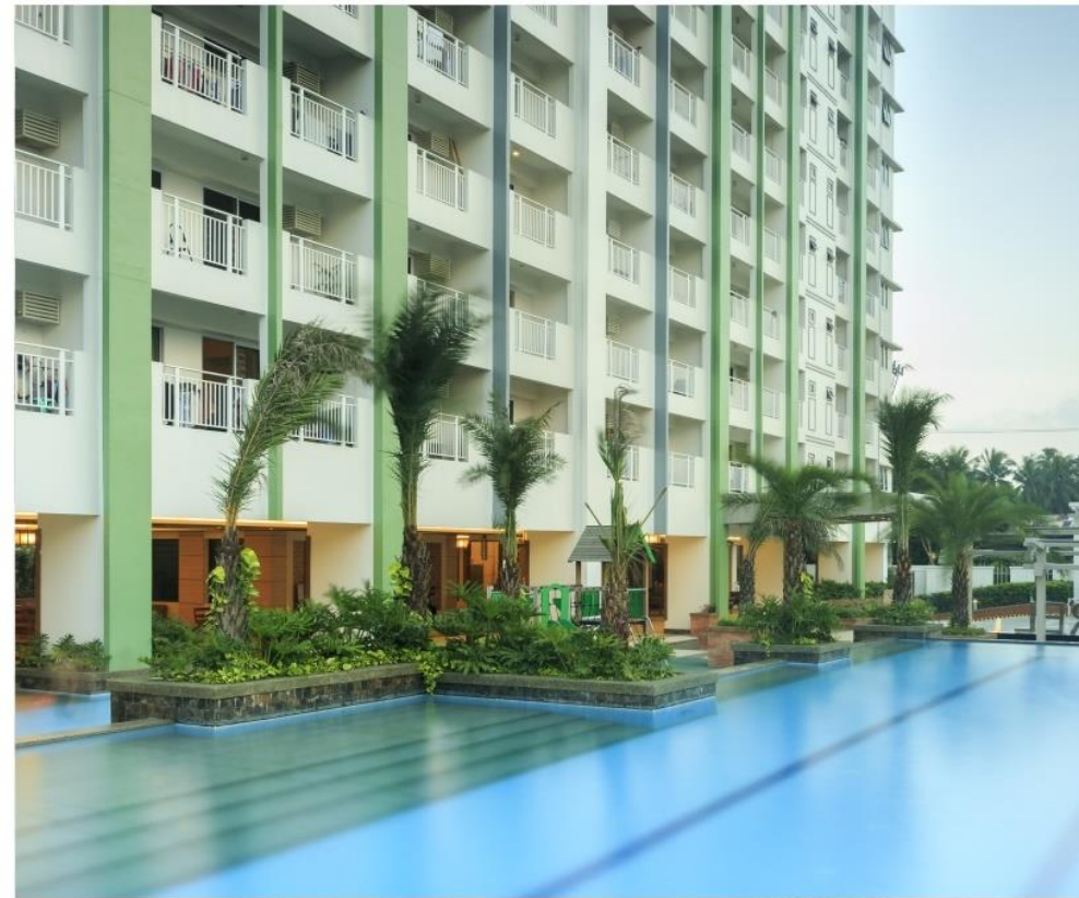
ACTUAL PHOTO OF THE DEVELOPMENT
