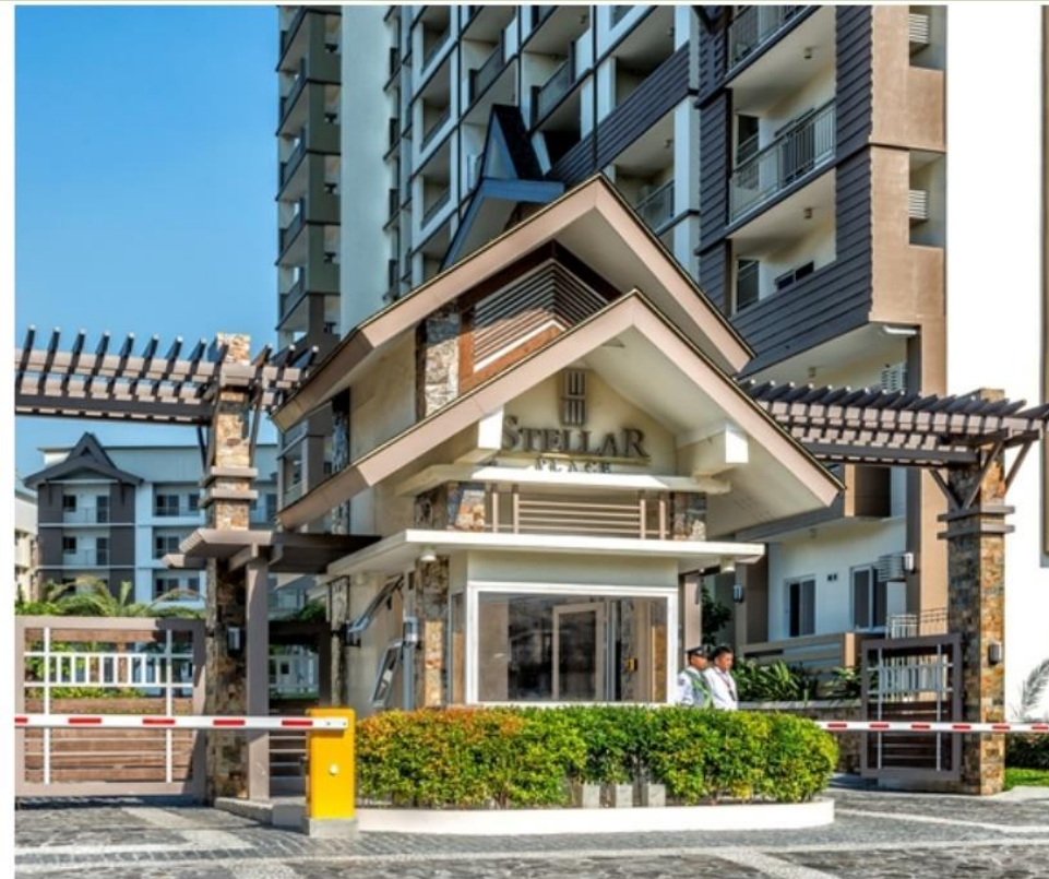
ACTUAL PHOTO OF THE DEVELOPMENT
